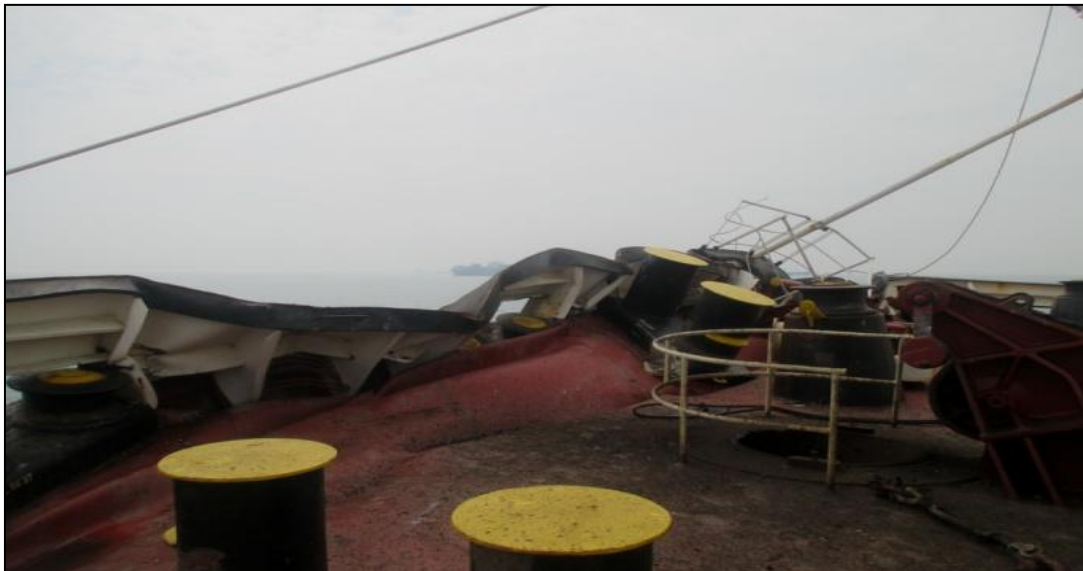
Figure 9: Bulwark and deck plating damage on the forecastle deck
